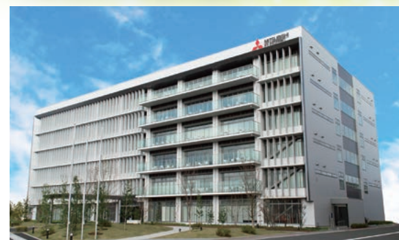
Air-Conditioning & Refrigeration Systems Works
